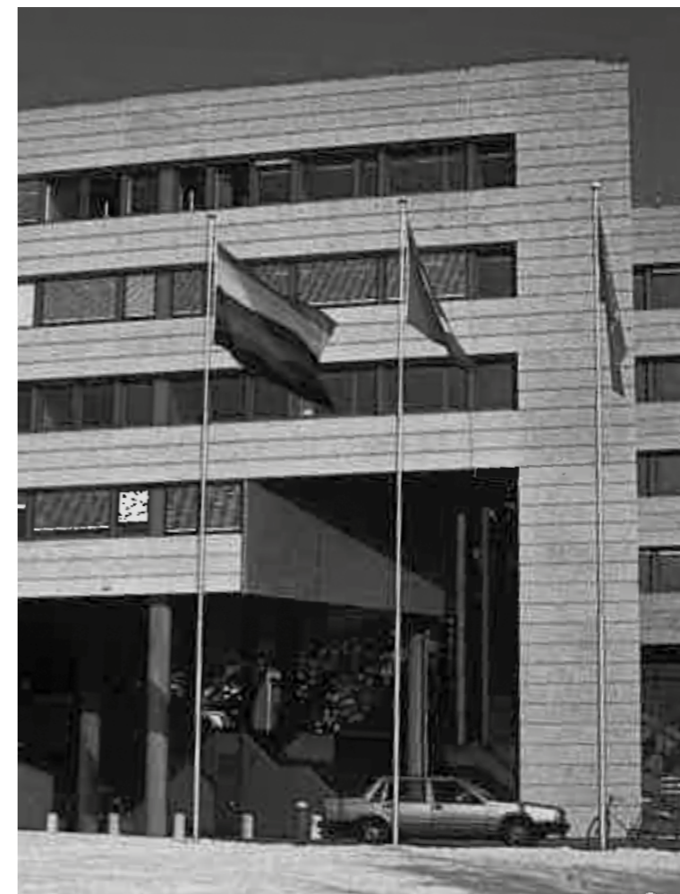
ICA Global Office Building in Geneva, Switzerland
